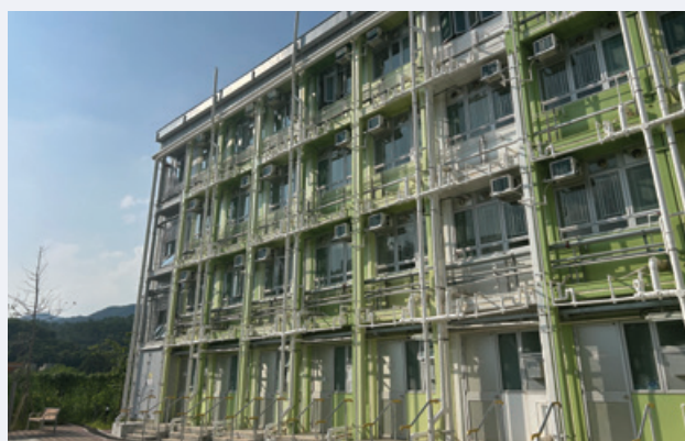
Lok Sin Village – the first reuse, recycling and relocation of MiC in Hong Kong
